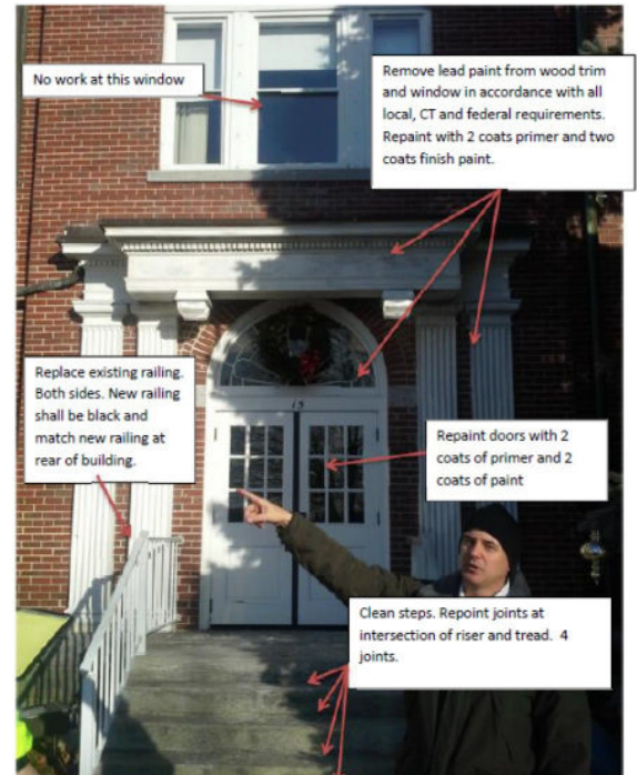
Waterford Front Entrance Work:
