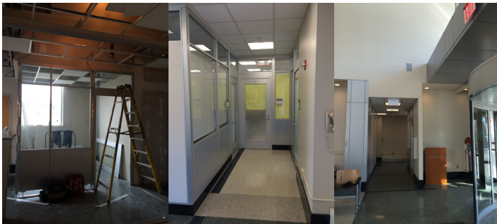
Figures 1-3. (Left) Before Photo; (Center + Right) Hospital call center after photos. Image credits: Gordian
